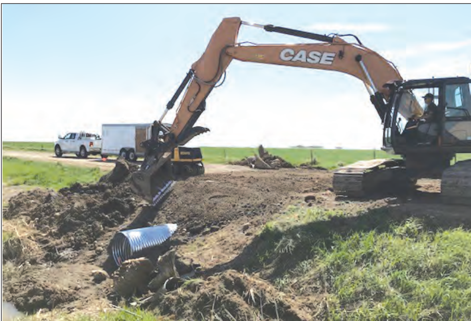
Culvert repair
