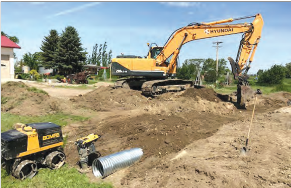
Culvert repair
