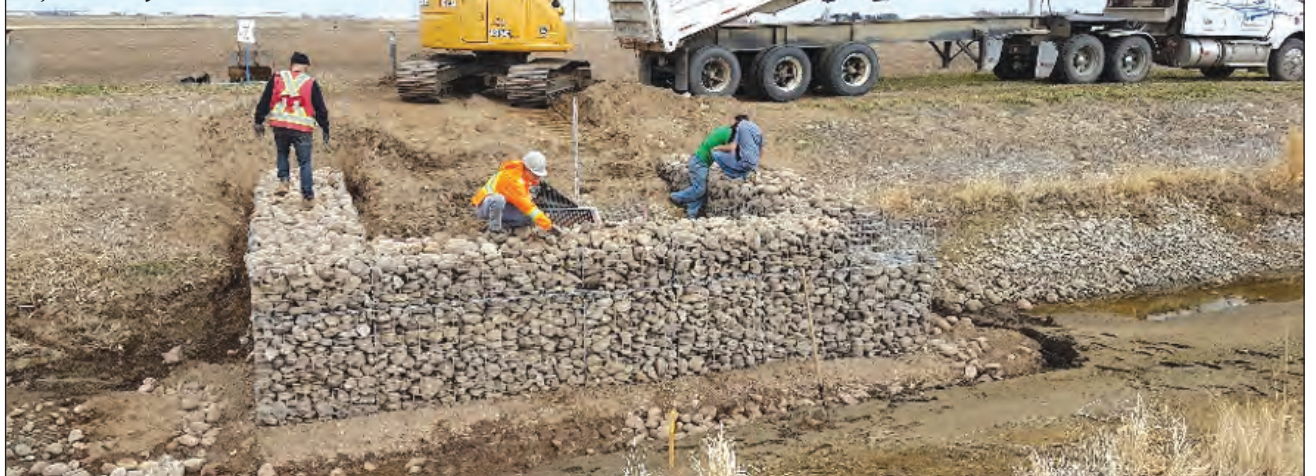
Filling Gabion Baskets for Infiltration System in TID
