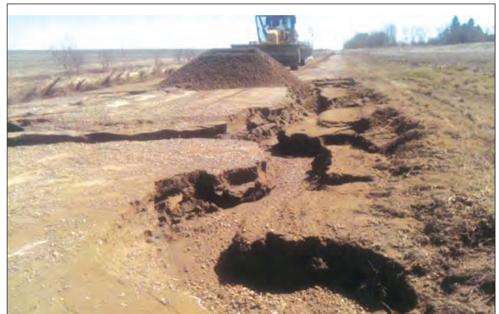
Temporaet road repairs
