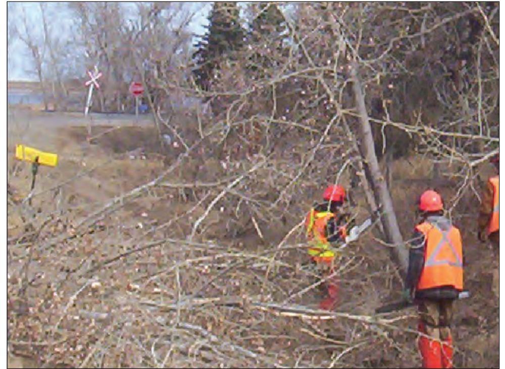
ASB staff clearing problem trees from a ditch
